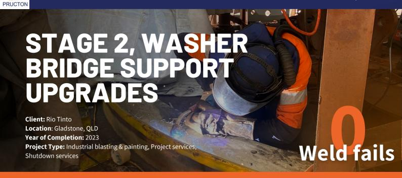
10km north-west of Gladstone, QLD sits Yarwun Alumina Refinery. Producing Alumina & hydrate, Yarwun refinery sees almost 3 million tonnes of alumina produced per year. To support this undertaking, Pructon was engaged to strengthen tank structures by replacing supporting members. These supporting members provide a foundation to support the centre tank top which in turn is supported off the walkways bridge above. The installation of these members has increased the safety longevity of the tank.
